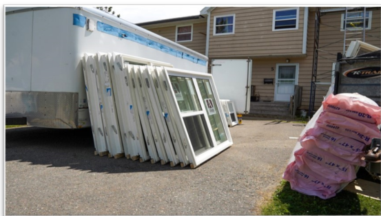
Spanish Bay home during construction
